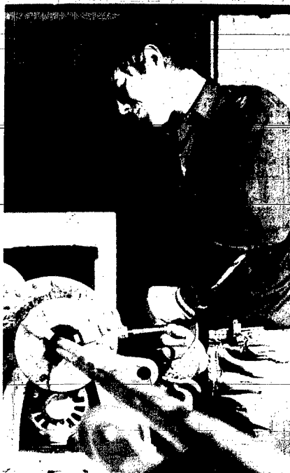
A WORKMAN from a Yankton plumbing firm cuts threads for part of the water line under construction at the one story medical center.
